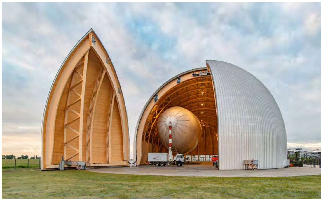
Pictured above & right: The Mülheim airship hangar in Germany combines innovation, sustainability, and a pioneering spirit to create a breathtaking piece of modern architecture. Copyright: Stefan Lamberty / WDL
