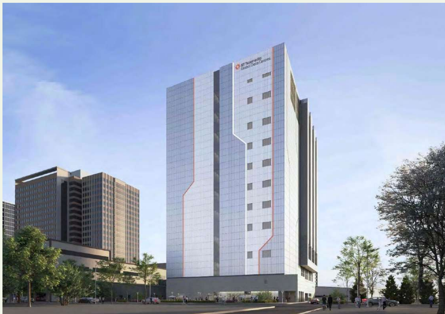
Situated within Gasan-dong, Geumcheon-gu, STT Seoul 1 is strategically located near Mokdong. The facility has convenient access to nearby sub-stations, as well as critical telecommunications, subway stations (Gasan Digital Complex and Doksan), logistics, and knowledge industry centres.
