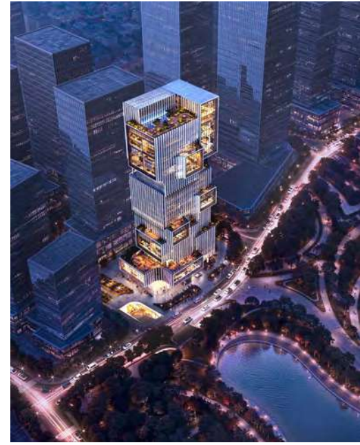
Portals and stacked volumes are illuminated at night, forming a lakeside landmark.
